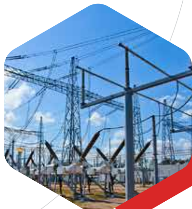
132KV Sub-Station Steel Gantry
